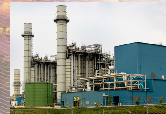
Zeeland Generating Station
