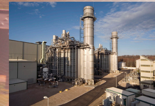
New Covert Generating Facility
